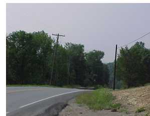
After slope flattening
